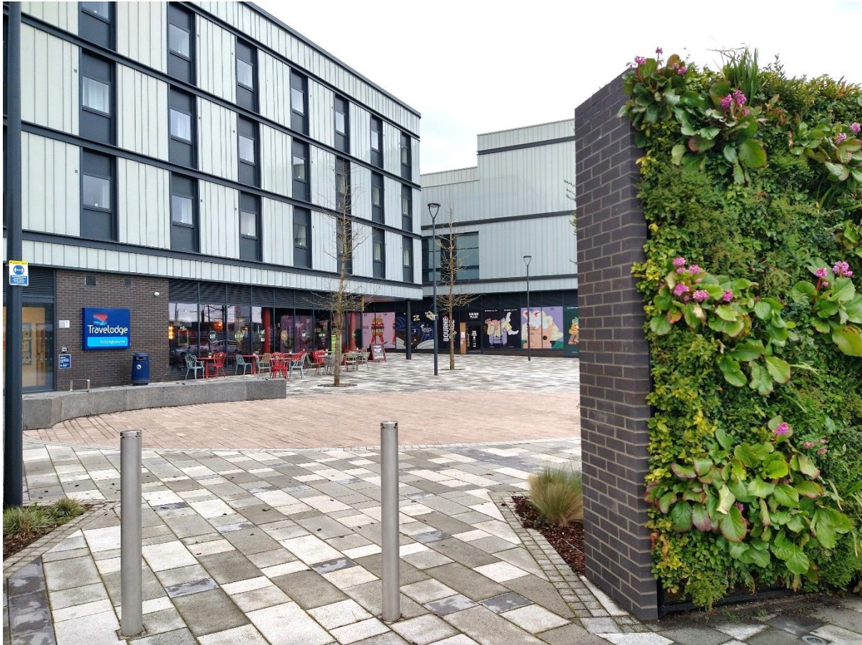
Bourne Place, part of the new connection between the railway station and the High Street
